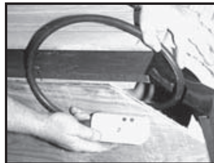
Ground fault interrupter plug & power cord fished through arched corner of the spa
