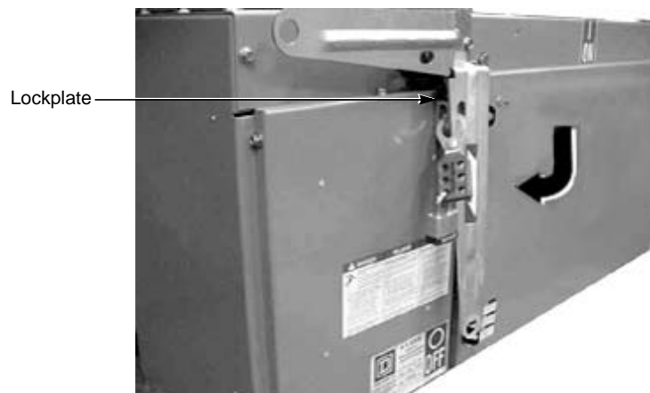
Figure 12 – Padlocking the Plug-In Unit Handle
